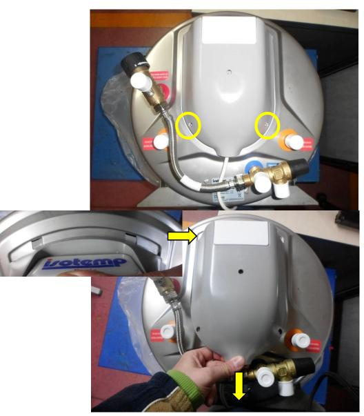
Remove the fixing screws of the cover
