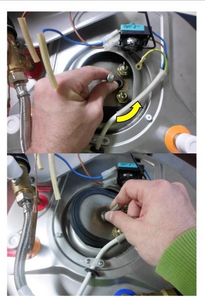
Rotate the bracket by 90° counterclockwise
