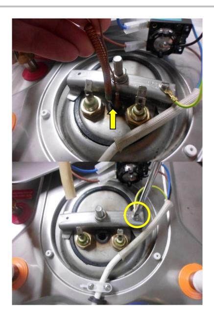
Remove the thermostat probes
