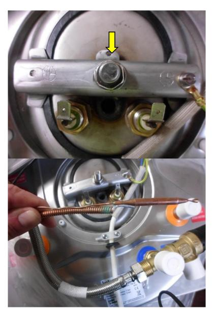
When reinstalling the bridge pay attention to the positioning, the part indicated by the arrow must be as in the picture or the hole for the thermostat probes will be covered.
