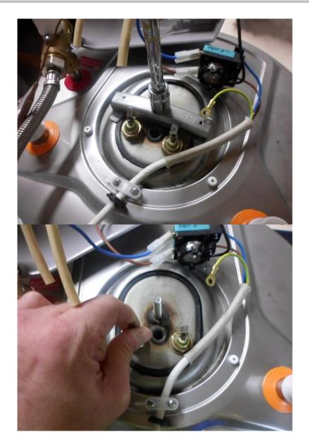
With a wrench pipe #14 remove the nut
